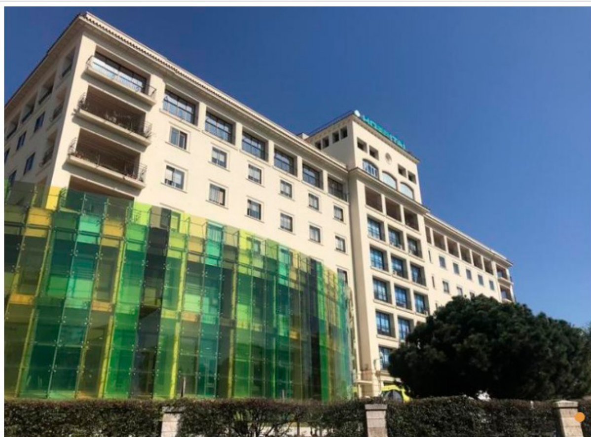
Hospital Regional de Málaga
